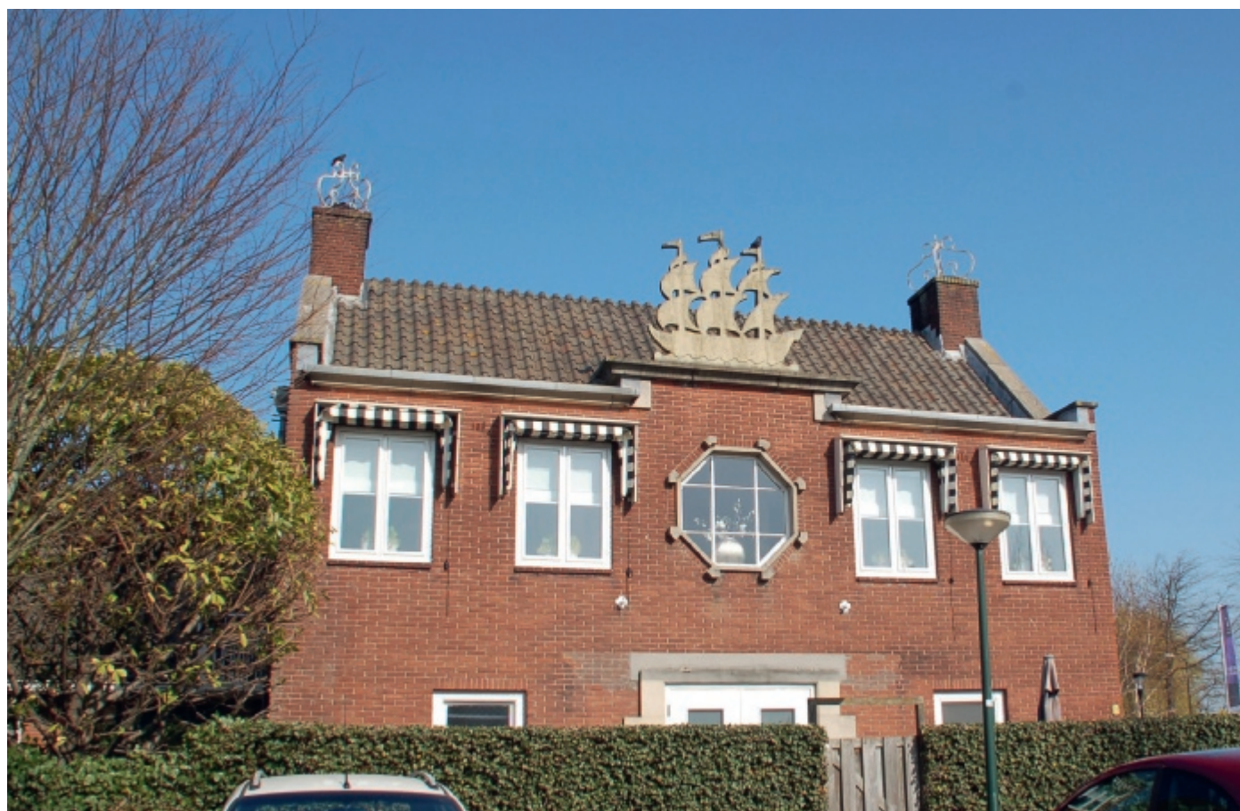
Merwestichting Hardinxveld-Giessendam. Architect: Sybold van Ravesteyn
